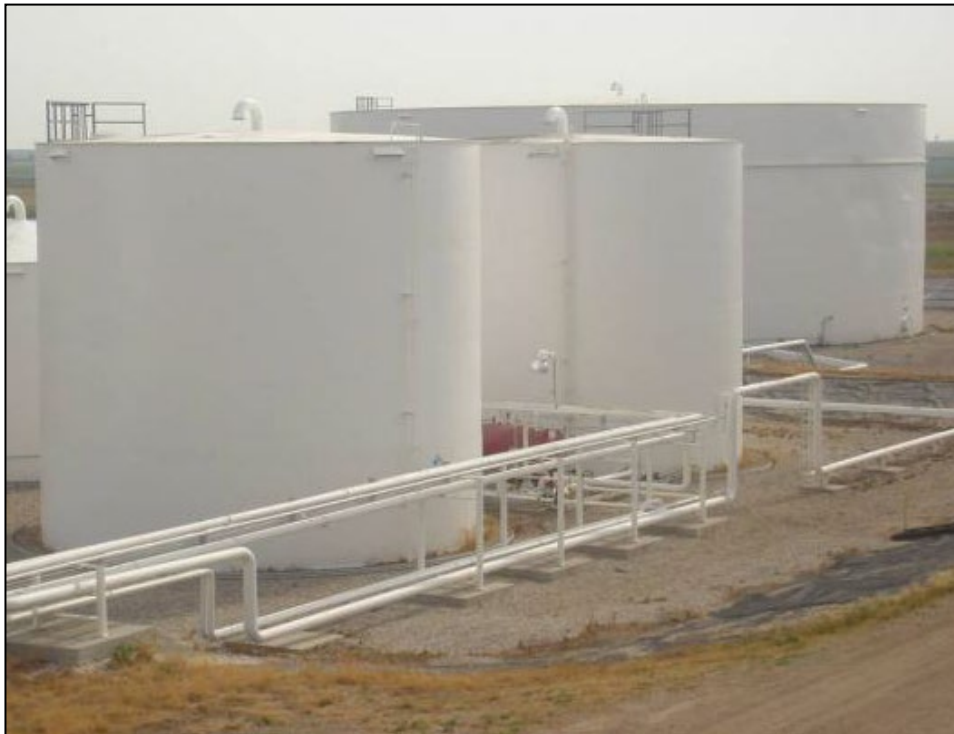
Figure 5.1: Internal Floating Roof Storage Tank
